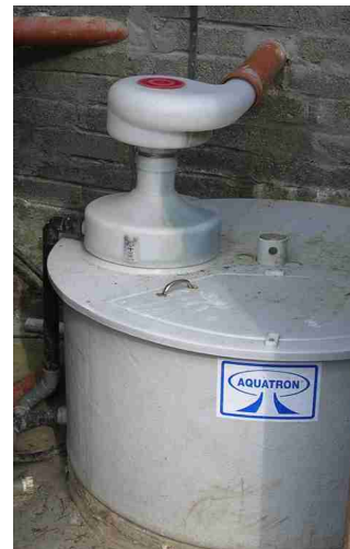
Aquatron faecal separator with rotating carousel for compost. Photo: Féidhlim Harty
