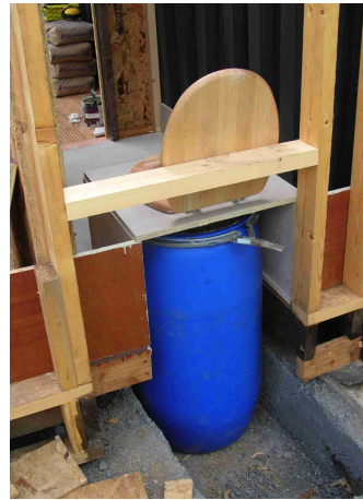
Front and rear photographs of low-tech domestic system. Remote composting semi-indoor use toilet, with large chamber which can be easily removed for maturation and then further composting as needed.
