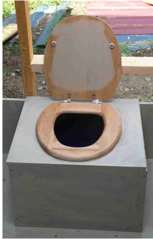
Front and rear photographs of low-tech domestic system. Remote composting semi-indoor use toilet, with large chamber which can be easily removed for maturation and then further composting as needed.
