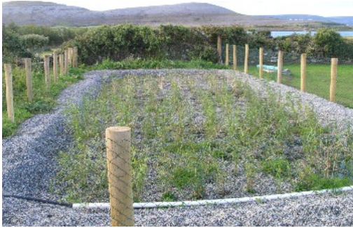
Newly planted reed bed system
